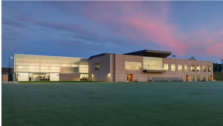
COMPASS MINERALS NPC (SPORTING KC TRAINING FACILITY) KANSAS CITY, KS
